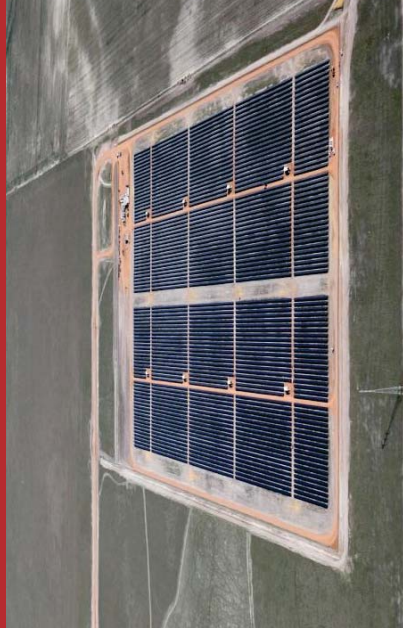
FIGURE 68: GREENOUGH RIVER SOLAR PV FARM, WESTERN AUSTRALIA SOURCE: GREENOUGH RIVER SOLAR FARM
