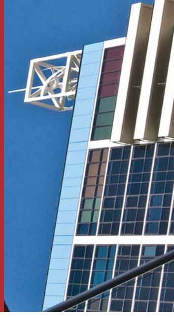
FIGURE 57: MICRO WIND TURBINE, INMARK TOWER, SYDNEY SOURCE: SYDNEY ARCHITECTURE
