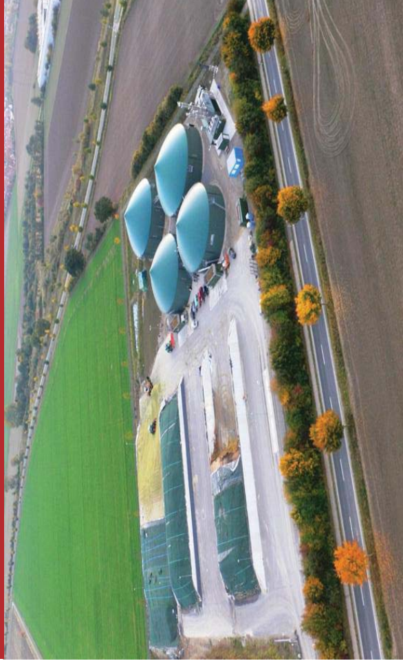
FIGURE 82: BIOGAS GRID INJECTION PLANT AT RONNENBERG FOR HANNOVER CHP NETWORK, GERMANY SOURCE: ENERGYCITY (STADTWERKE HANNOVER AG)
