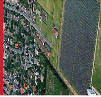
FIGURE 8: MARSTAL DISTRICT HEATING
